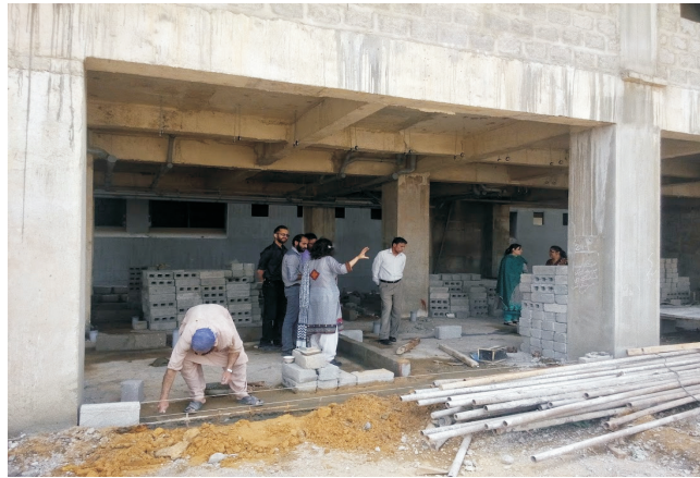
The foundation must be sound: Dr. Moazam in action
